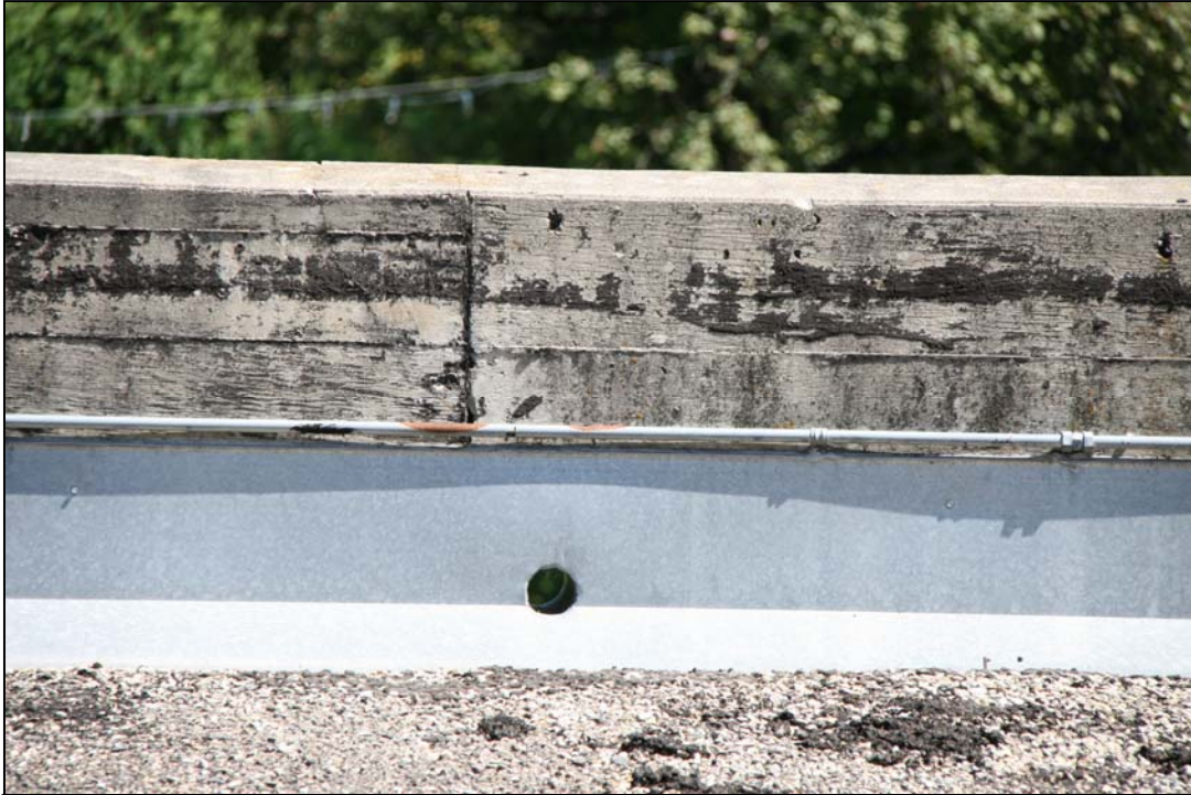
Photo # 13 This photo shows a view of the typical overflow scupper.
